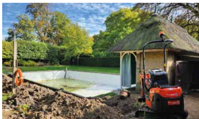
Improvement works begin on the bathing pool
