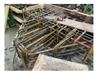
GA to try to avoid hitting the reinforcement when installing the anchors to the temporary props. SaW confirmed that the 32mm diameter bars are critical for the integrity of the corbel, however the 25mm bars (at the face to the prop) are less so.
