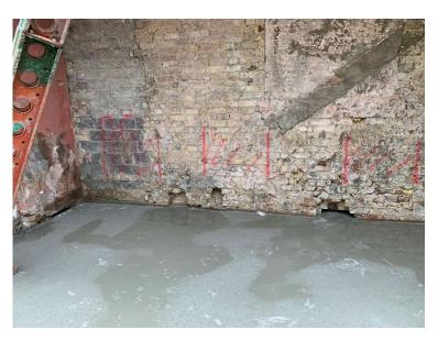
Complete the work as agreed but pay close attention to any brickwork being removed. If a brick is locked in place but the surrounding bricks are loose, do not remove the wedged brick.
